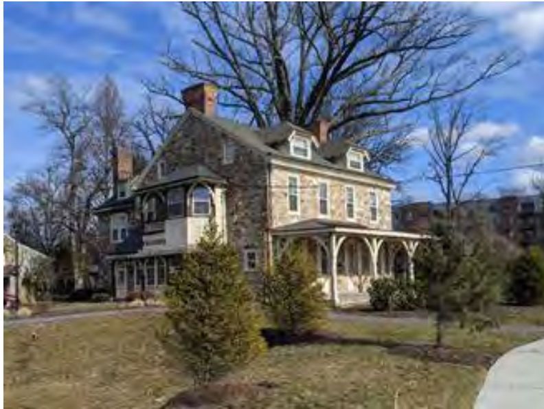
Ivy Cottage (205) constructed c. 1800 by Colonel Richard Thomas (III) (Commonwealth 2021).
