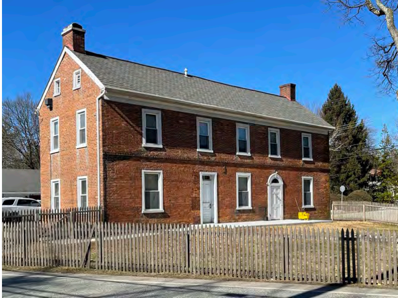
William Everhart's brick store house (046) (Commonwealth 2021).
