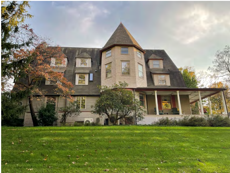
Francis W. Kennedy House (143). Designed in 1889 by renowned architect Frank Miles Day as a summer cottage in Bradford Hills (Commonwealth 2021).
