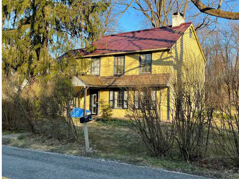
David Ashbridge Log House (021) constructed in 1782 (Commonwealth 2021).
